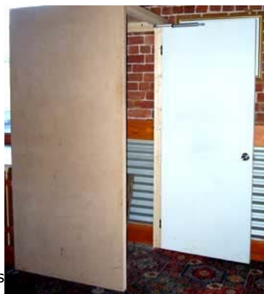
Example of a lockable barrier around a trapdoor in a public area.
