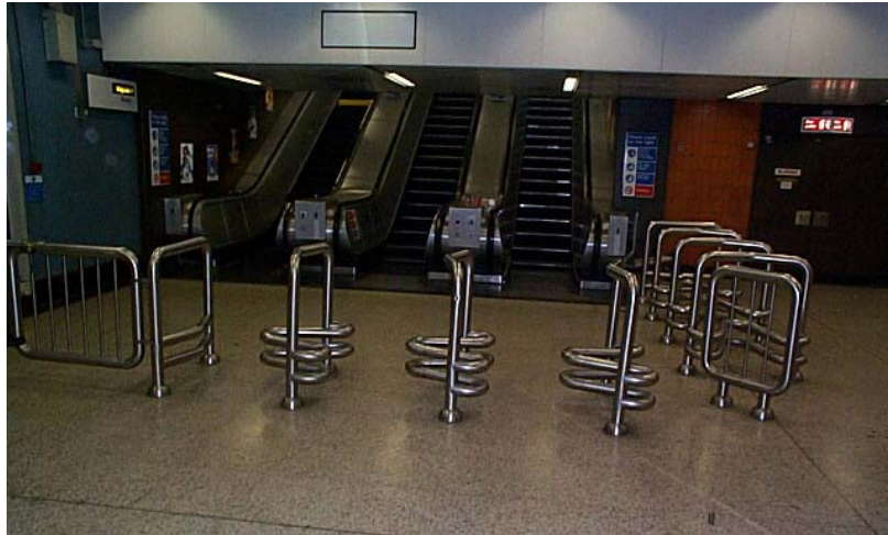
Barriers at Heathrow Airport to prevent trolleys being taken onto escalators.
