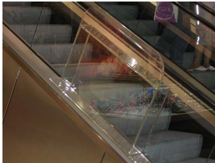
Example of an escalator guard designed to prevent travel up the outside.
